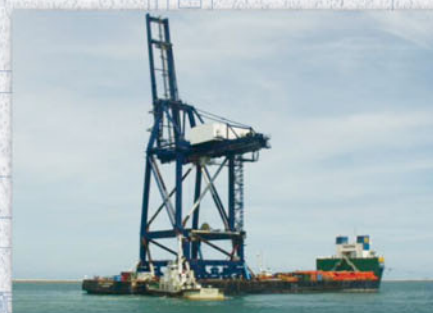
Specification, acquisition, delivery and installation of all equipment for the terminal
