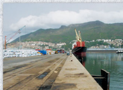
Before: A conventional multi-purpose port
