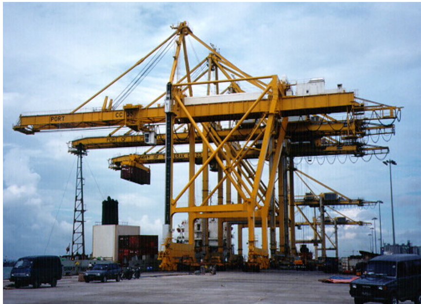
Hitachi Crane in Surabaya, Indonesia after Span Change (18 metres)
