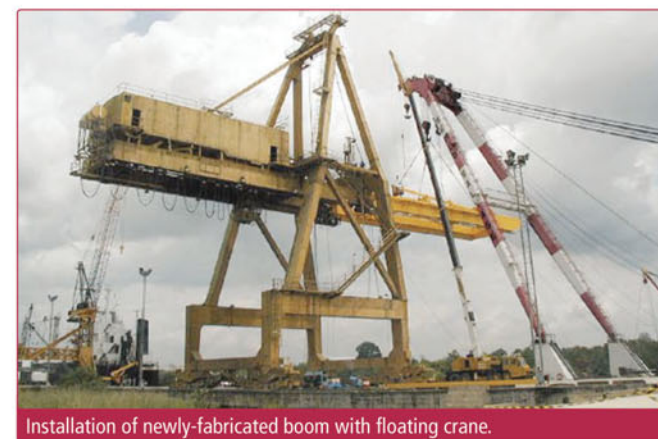
Installation of newly-fabricated boom with floating crane.
